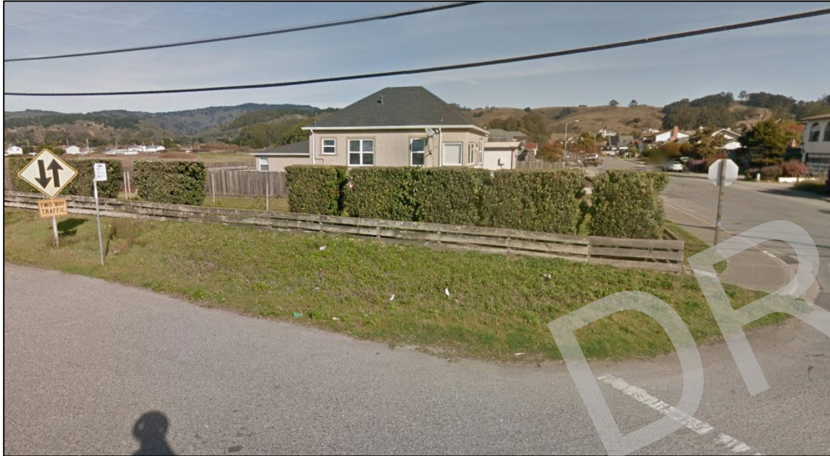
Current sidewalk gap at Terrace Avenue bus stop
