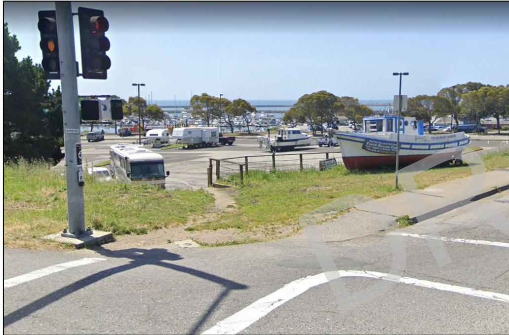
Existing curb at Highway 1/Capistrano Road
