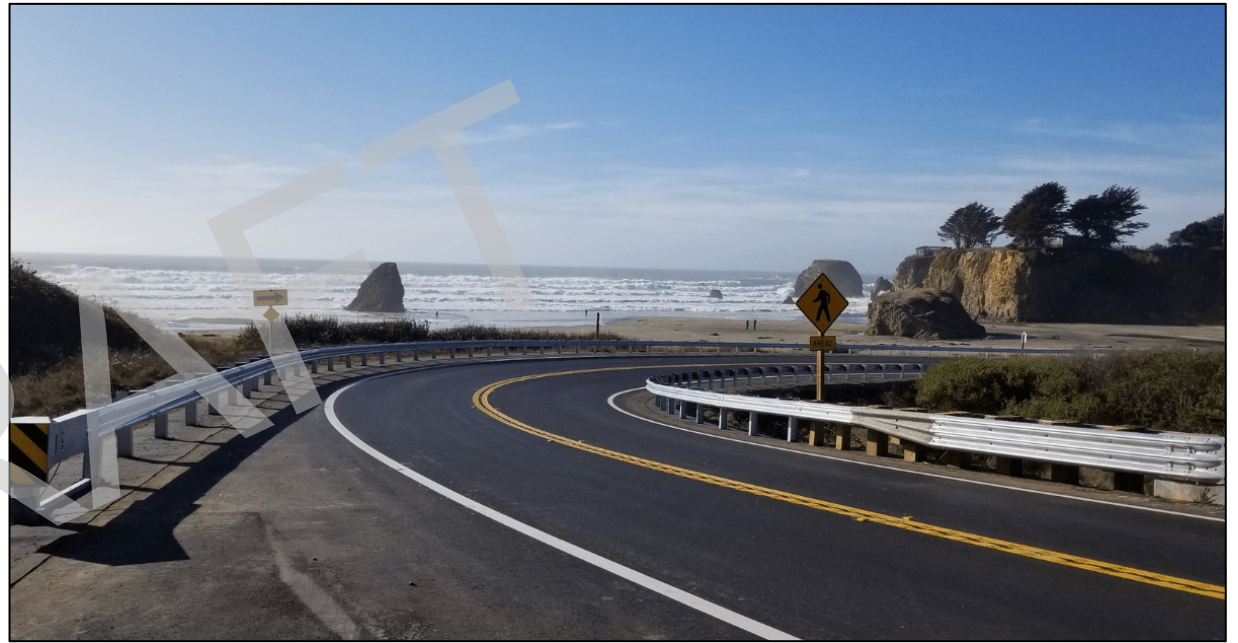
Recent Caltrans Highway 1 Project in Mendocino County
