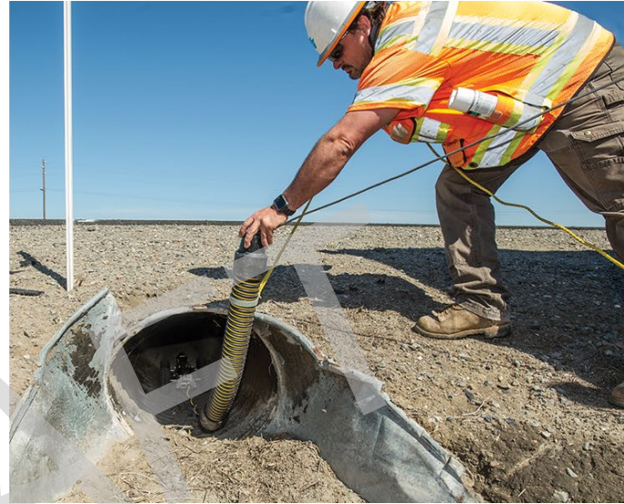
Robotic Culvert Inspection
