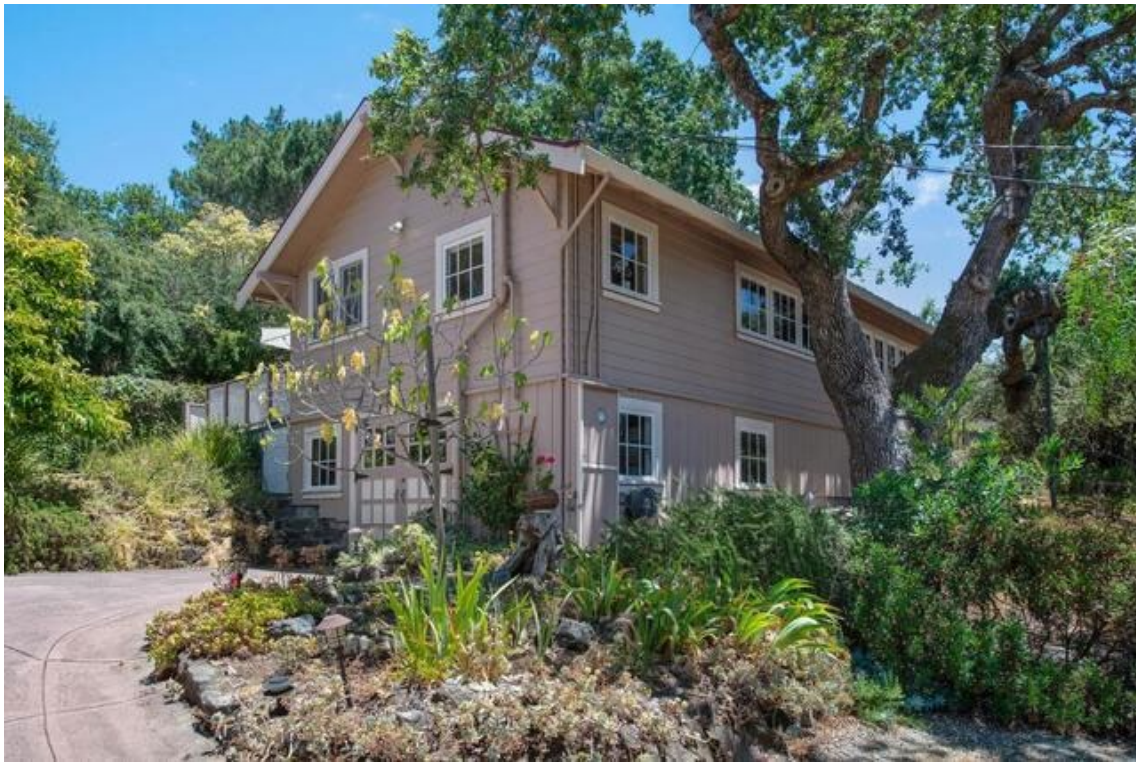
Photograph 1 890 Upton Road View: Front end of the building facing the street and side façade. This appears to be the older section.
