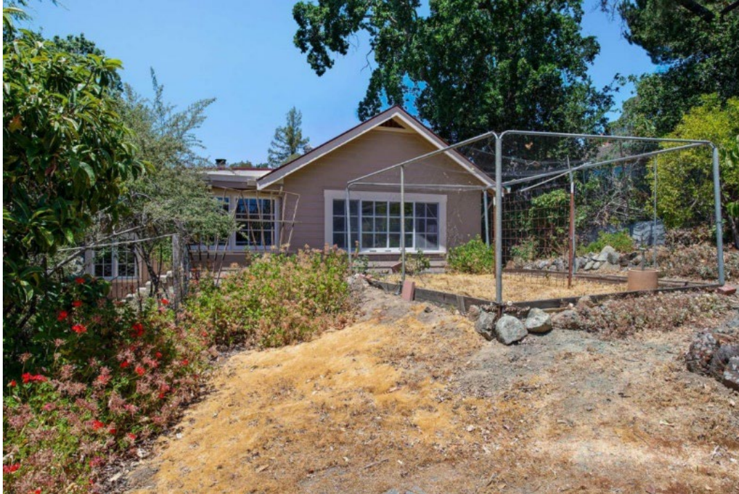
Photograph 7 890 Upton Road – Rear of the house, showing the back of the side addition.
