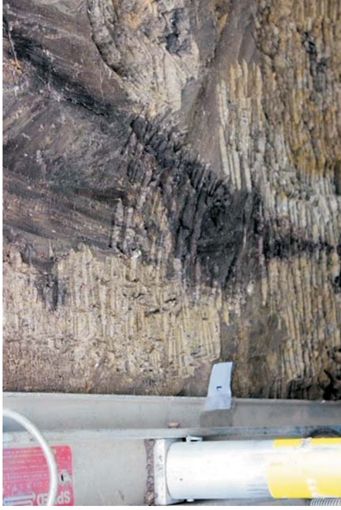
Fault trace at Shore #1
