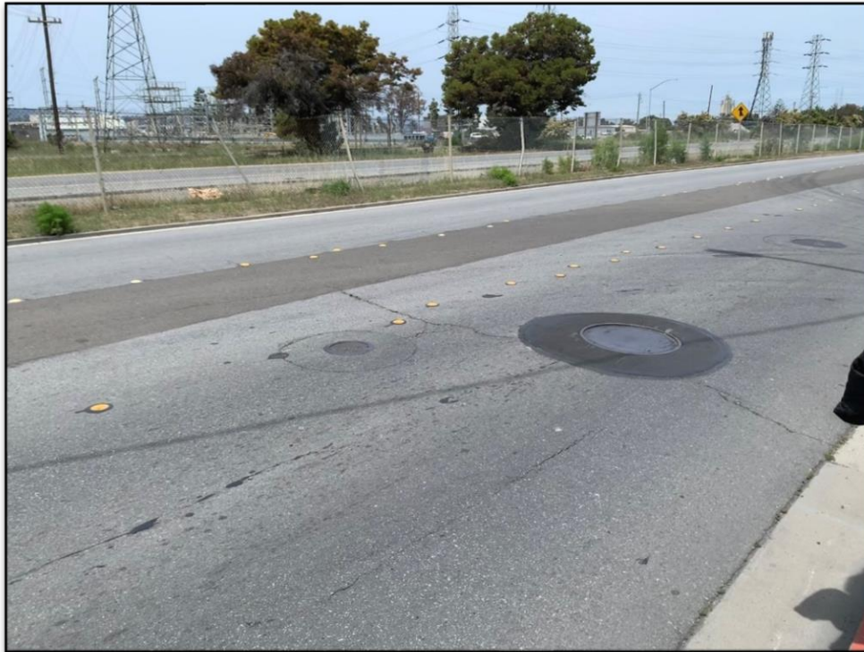
Photo 6. View west of Segment 3 across Bayshore Road and Seaport Boulevard.
