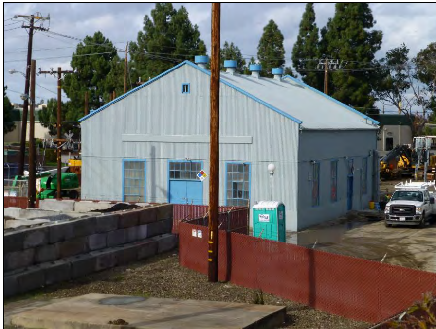
Photograph 4: South and east side of control house, camera facing northeast, December 16, 2014.
