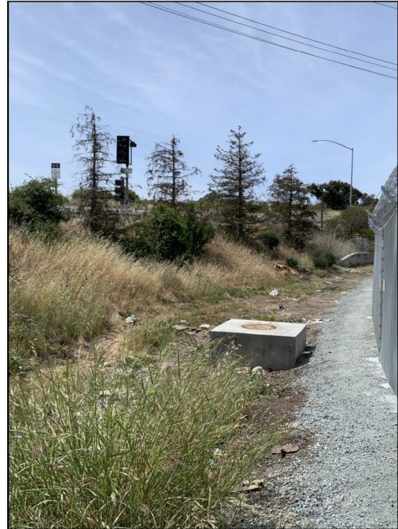
Facing southwest with view of Manhole 3629.
