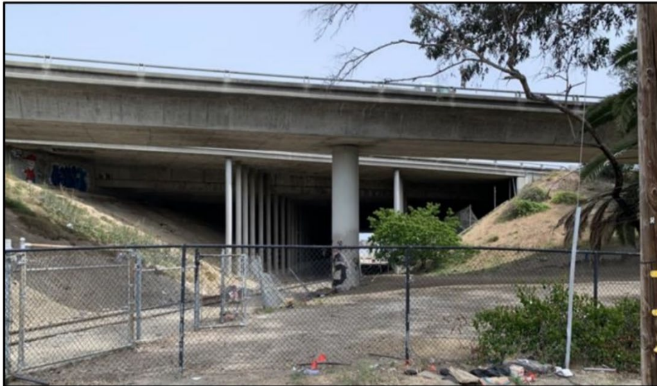
Facing northeast from the County lot. View of the US 101/Woodside Road offramp in the center and US 101 underpass in the background.
