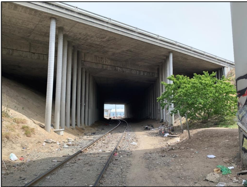
Photo 2. View northeast of Highway 101 underpass near western end of Segment 1.
