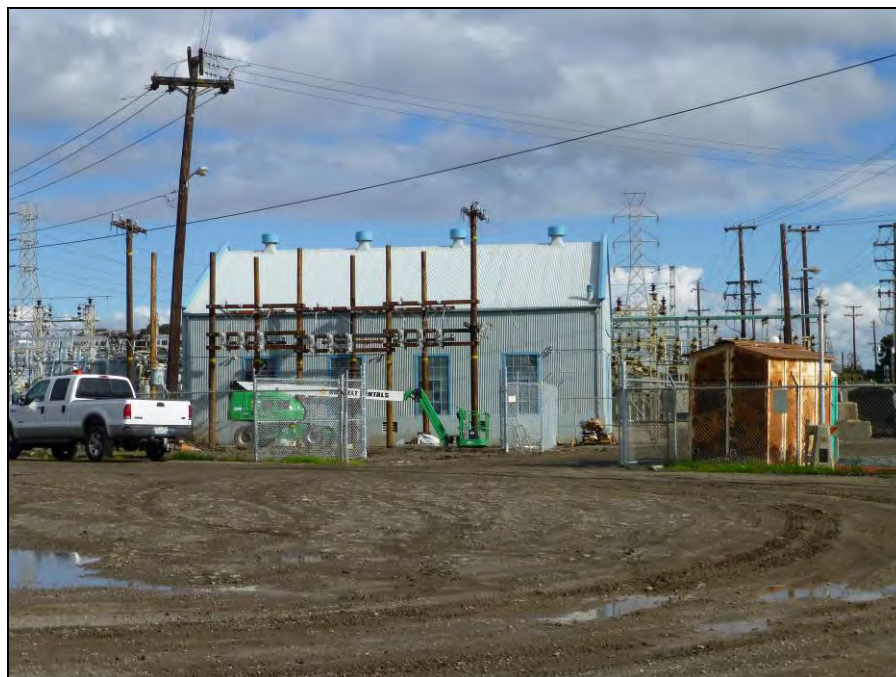
Photograph 5: West side of control house, and shed, camera facing east, December 16, 2014.
