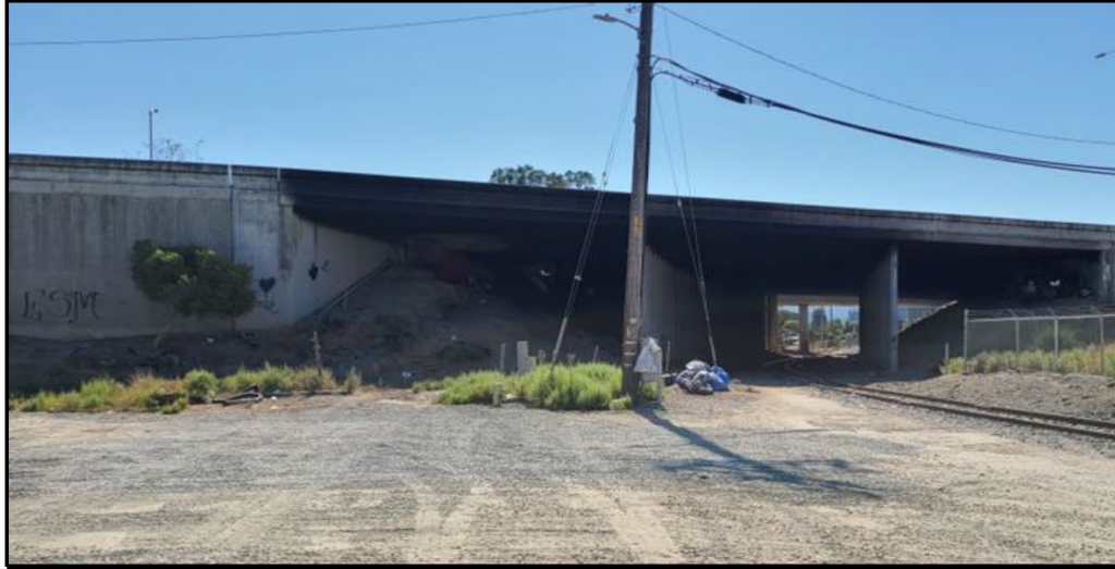
Facing southwest near the entrance of the PG&E Substation. View of US 101 underpass and UPRR track.
