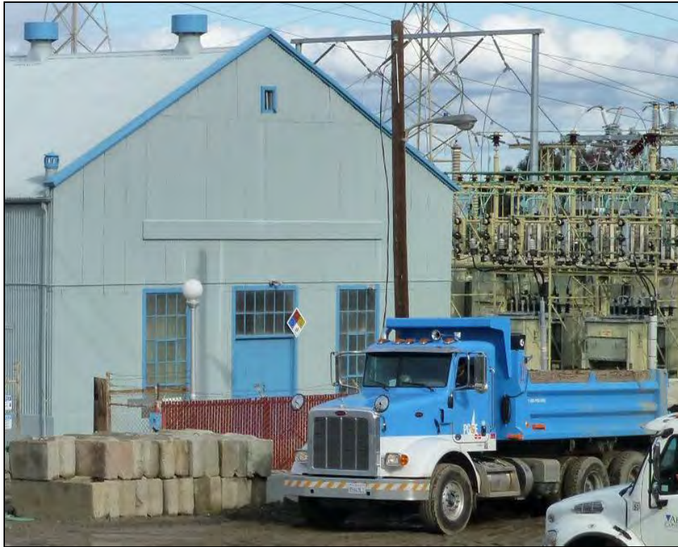
Plate 2: 2014 photograph of south side of Redwood City Substation control house (JRP).
