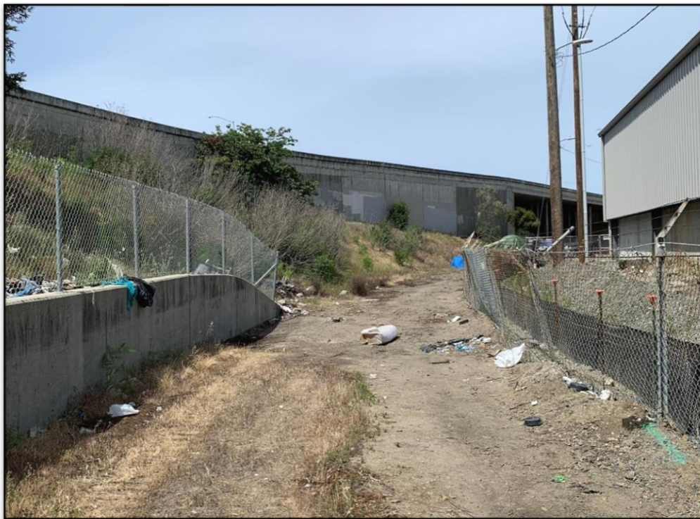
Photo 4. View west toward the Highway 101 underpass near the western end of Segment 2.
