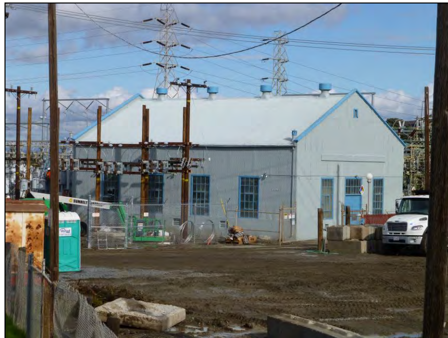
Photograph 3: South and west side of control house, camera facing northeast, December 16, 2014.
