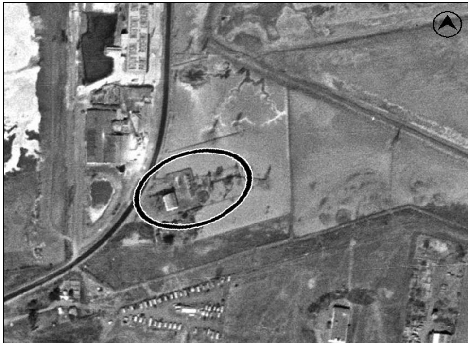
Plate 3: Pre-freeway 1948 aerial of Redwood City Substation. 9
