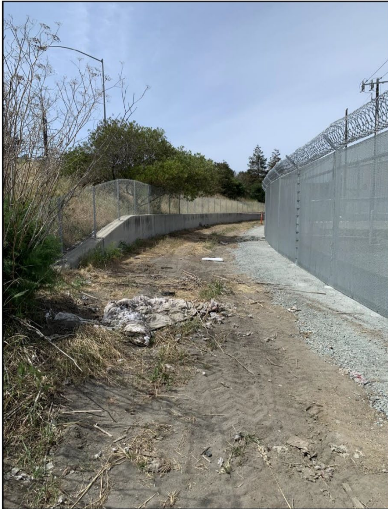
Facing west from Manhole 3628. Note the retaining wall supporting the US 101/Seaport Boulevard onramp on the left and the PG&E Substation fence line on the right.
