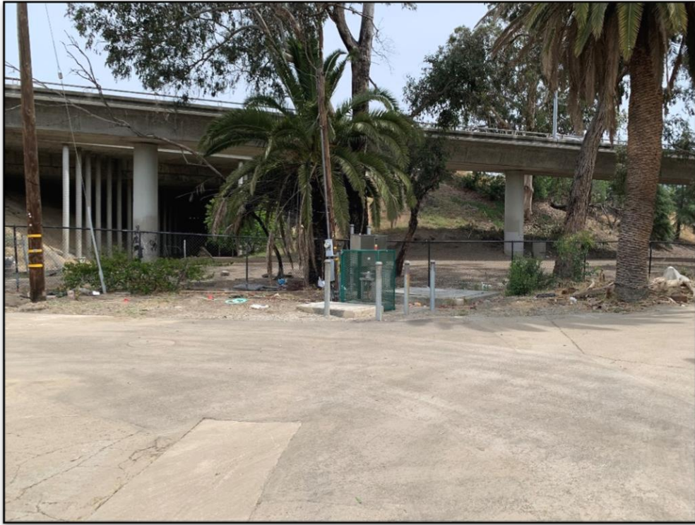
Photo 1. View north from staging area in Segment 1, south of Highway 101 off-ramp.
