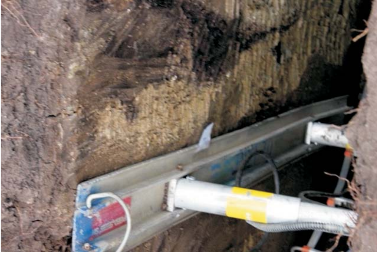
Fault trace at Shore #1
