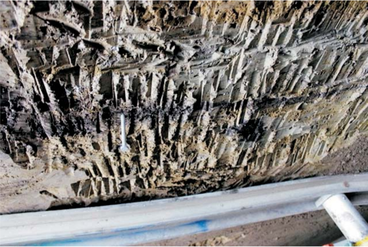
Fault trace at Shore #1
