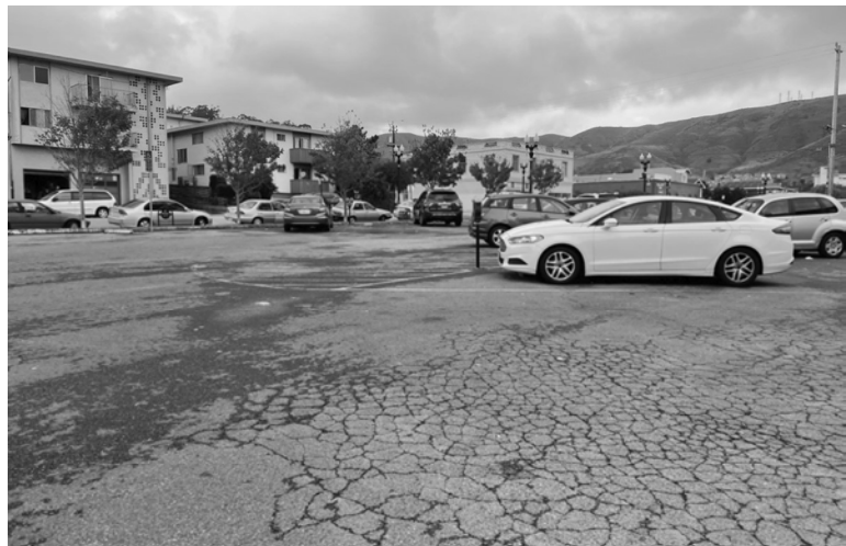
616 Linden Avenue – Southeast Corner – Direction is Northwest
