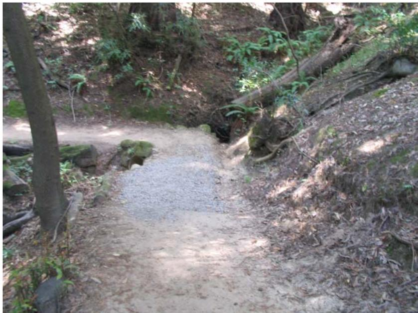
*View from along Bear Gulch Trail, showing recent repair and reconstruction of the trail due to erosion and trail failure repair included new trail with aggregate base material and the installation of a new small drainage culvert and rock riprap at the swale.*
