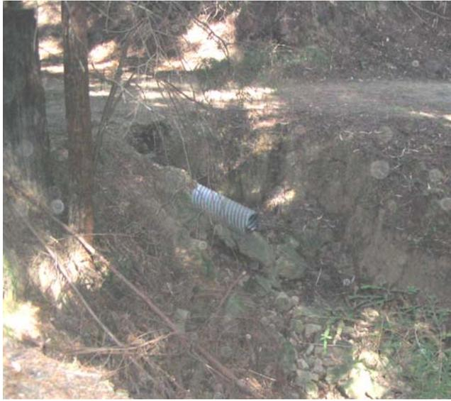
*Erosion occurring at Culvert crossing along Loop trail on the way up to Salamander Flats.*
