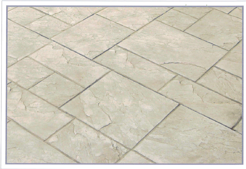
STAMPED CONCRETE DRIVEWAY AND PATIO FINISH
