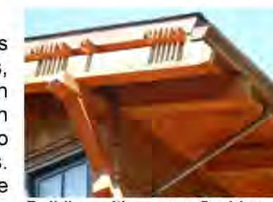
Building with copper flashing, gutter and drainpipe.
